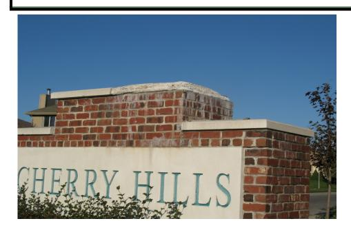
Here are two pictures of the entrance sign on 107th and Redick where one of the four top caps is starting to deteriorate. This appears to be the only case of this happening in Cherry Hills. Upon investigating the cost of this repair, it was discovered that these caps are specially made. The cost estimates to repair this one cap was in the neighborhood of \$800.00. There are roughly 14 of this size caps and roughly 60 larger caps at the other 5 entrances.
